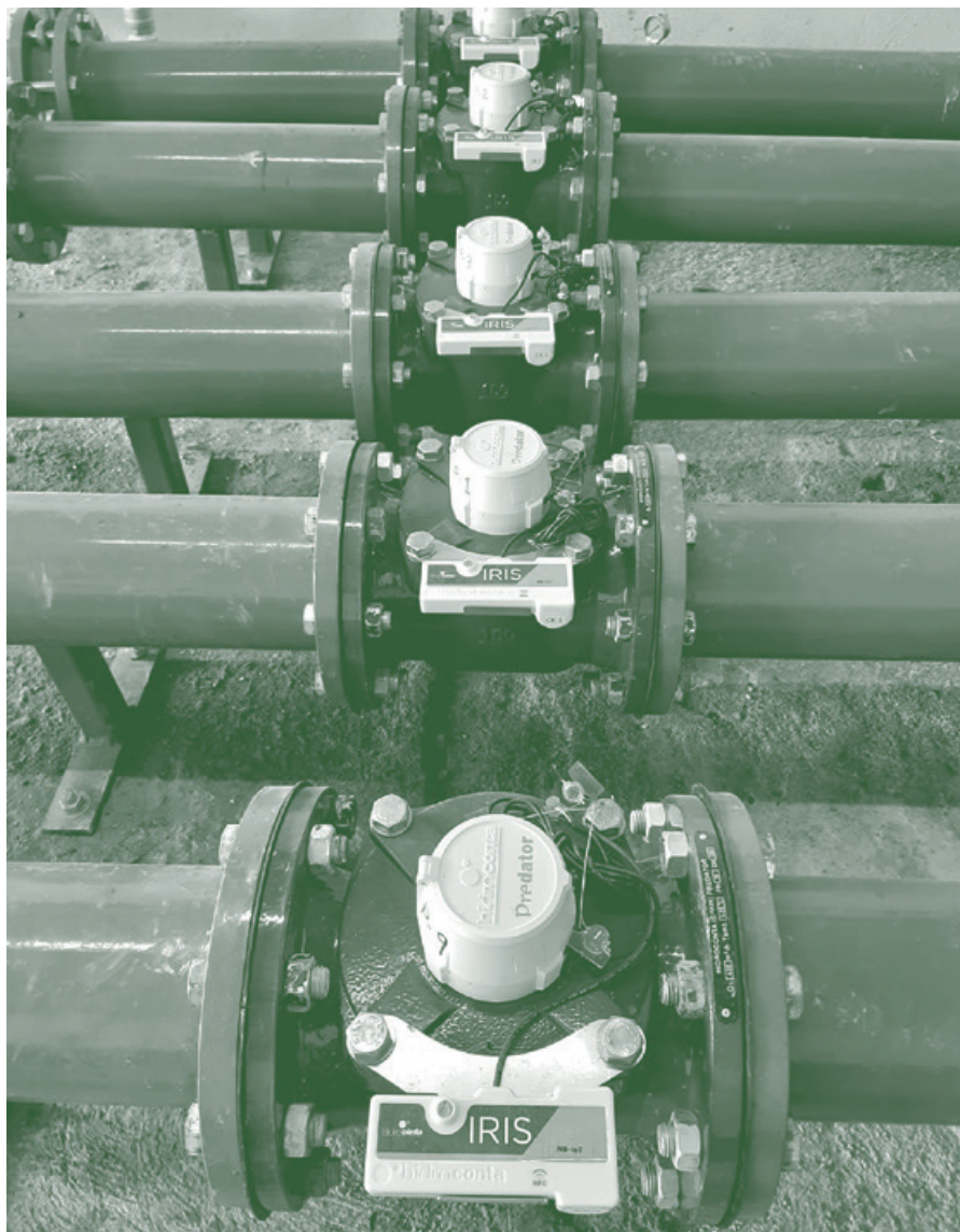
Digitized water meters with Iris at the Irrigation Association Consortium Cota 400
